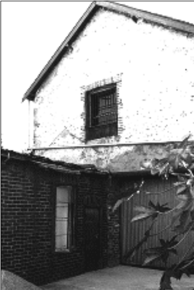
Figure 14: The flashing line of the former Stable roof was evident on the rear wall of the warehouse
