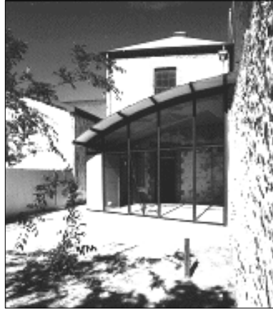
Figure 13: The addition of a modern and sympathetic conservatory provides required living space
