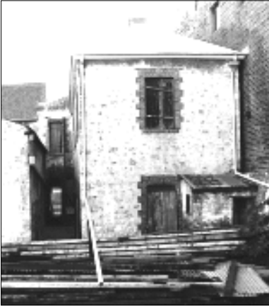
Figure 12: The rear to the former Residence in 1986
