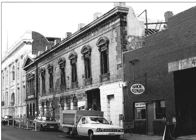
Figure 1: The Moores Building facade in 1986
