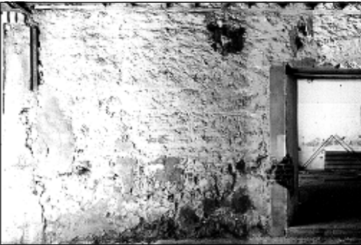
Figure 20: One of the walls which were used to anchor the facade
