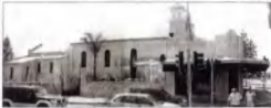
• The old synagogue site on Perry Street (see South Terrace) is Fremontle's historic heritage area.
