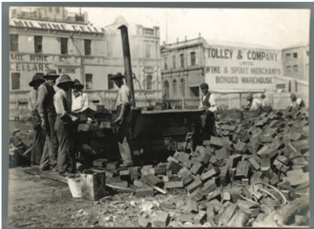
Pioneer Park Fremantle. Cleaning jarrah street blocks for re-use in September 1905, just months after tramlines began to be laid throughout Fremantle. From John Dowson's Old Fremantle .
