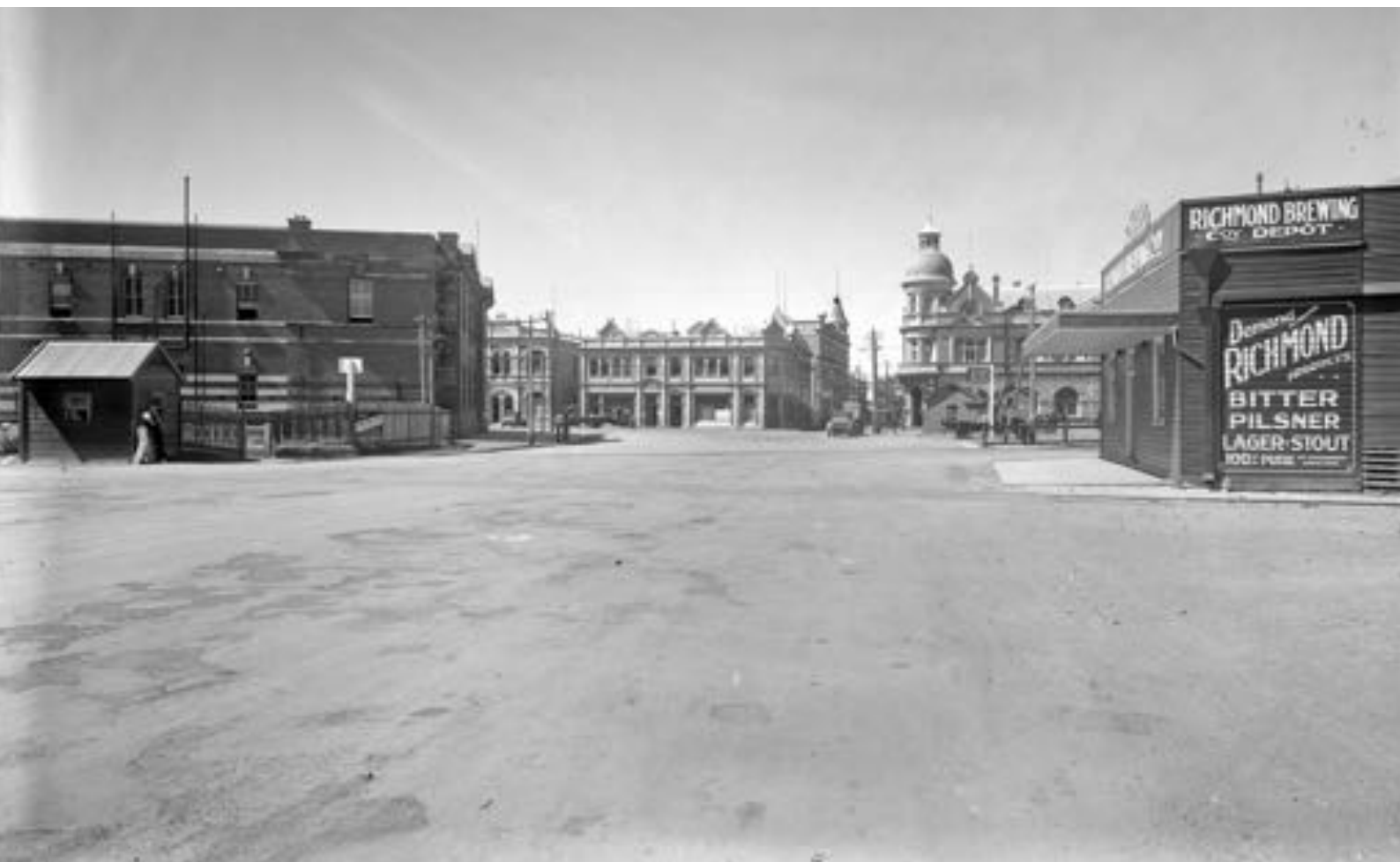
Top: Soon after being laid, wooden blocks are pulled up for the laying of tram tracks in 1905, here corner of High and Cliff Streets. Bottom: The extensive use of wooden blocks, put down here in 1911, can be seen on the left under the bitumen in this 1934 image of Cliff Street looking south to the entrance of the town at Phillimore Street. The 1907 Customs House on the left, brick and stone built using WA hardwoods, replaced Fremantle's first railway station. On the right is the brand new Richmond Brewing Depot, corner of Fleet Street, with capacity for 2,500 18 gallon casks, or 45,000 gallons of refrigerated beer, all shipped from Melbourne.
